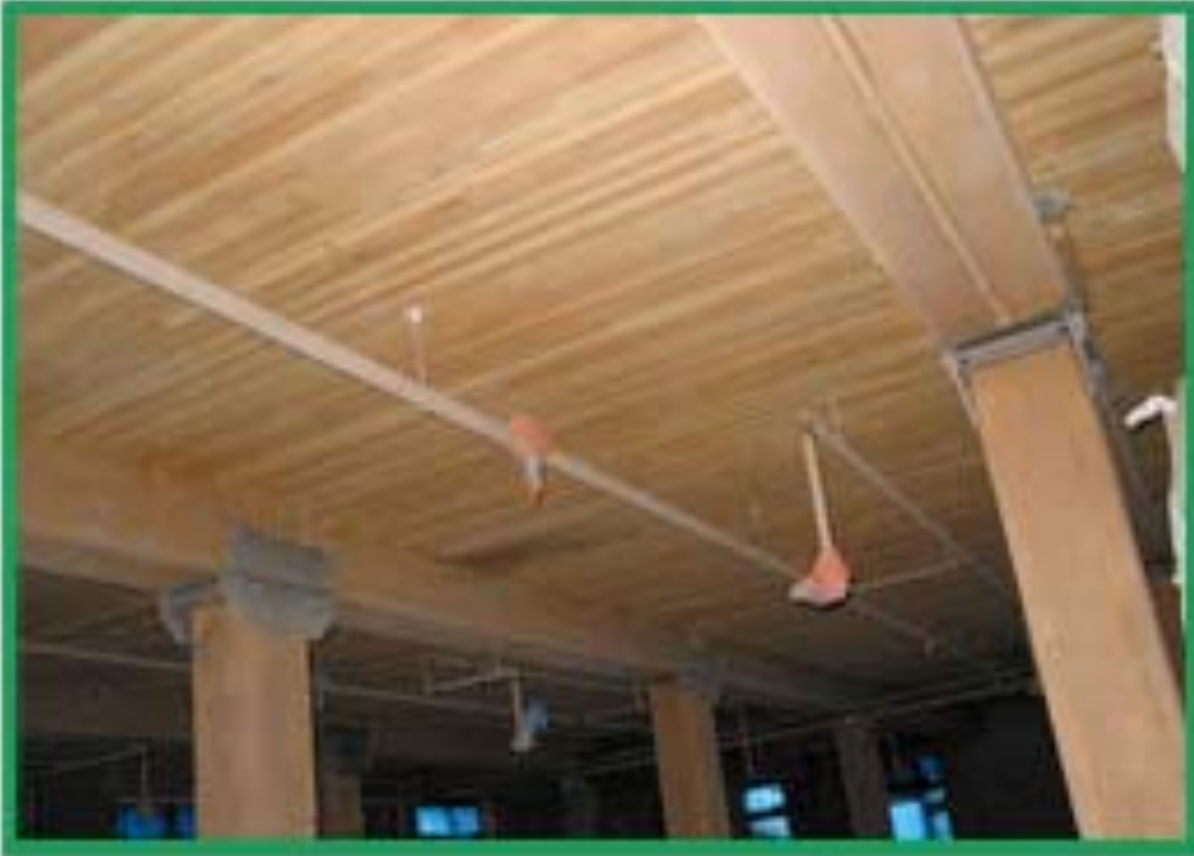
Results of glass-bead blasting on ceiling, beams and columns, August 2007
