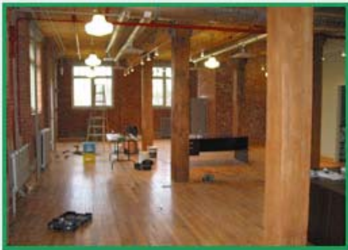
CMLC Lobby Area nearing completion, Sept 2007
