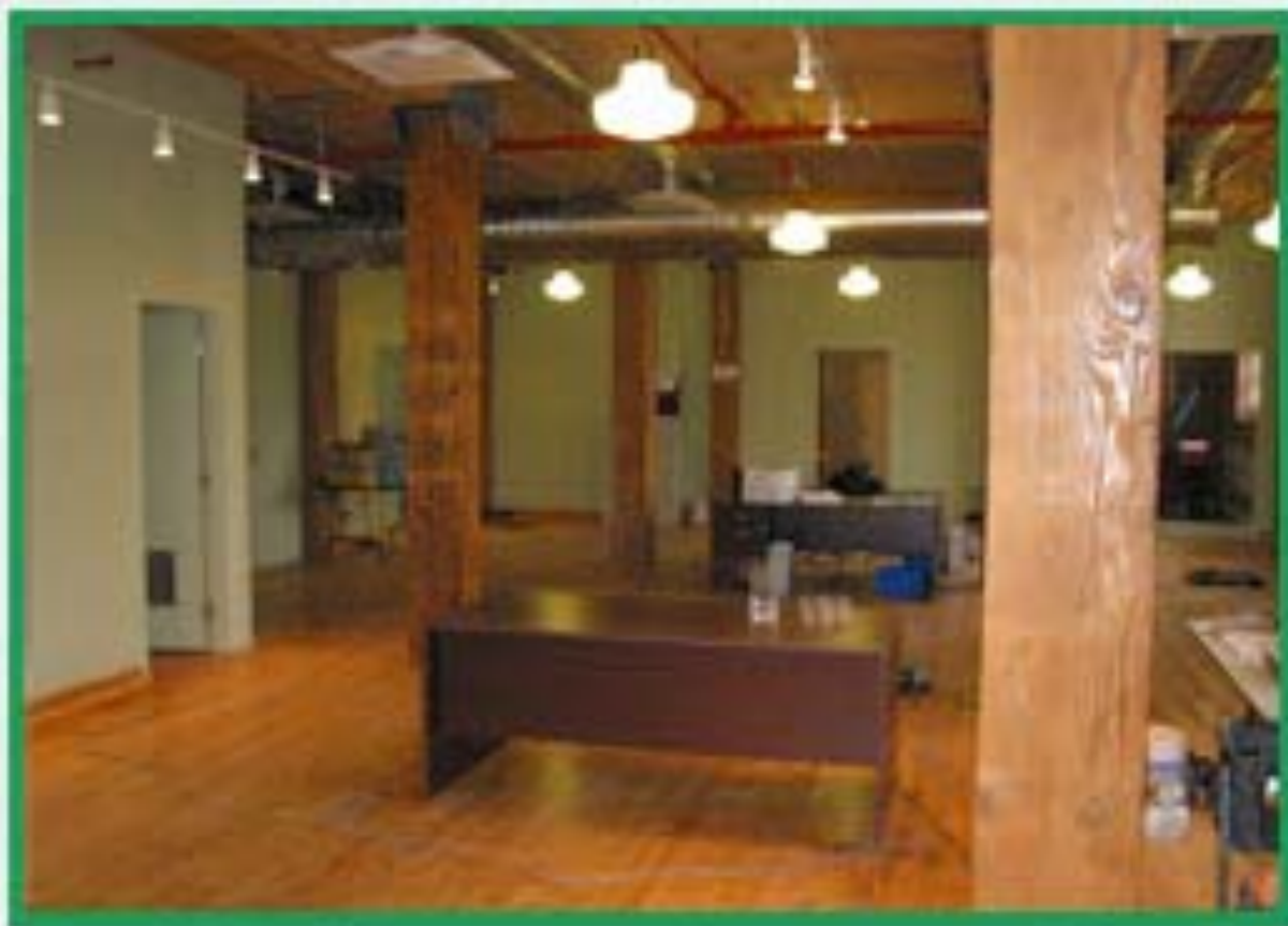
CMLC Staff Area nearing completion, Sept 2007
