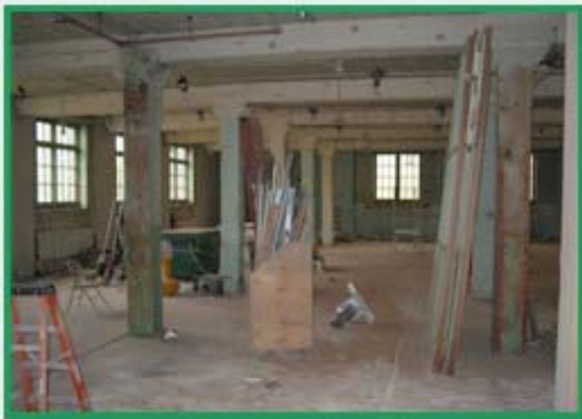
Before blasting old paint off, August 2007
