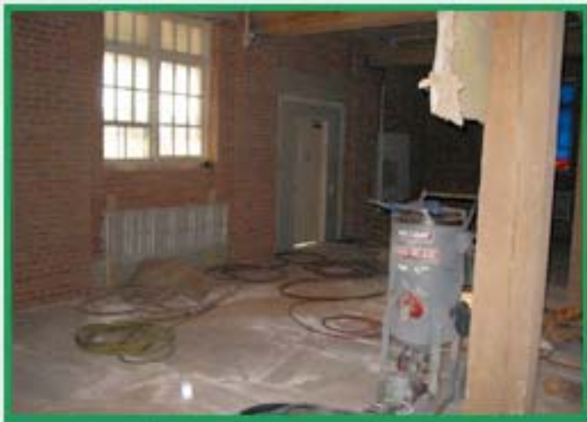
Results of blasting on brick interior, August 2007
